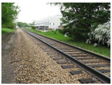
The concept of railroad ballast has much to do with tie support and drainage of water from contact with ties. On the support side of the equation we find that ties hold the track in place vertically and horizontally. To that end the ties must be trapped in somewhat an inflexible but elastic membrane of stone. Crushed stone is typically used for the purpose. The angular faces of modest size stones lock the tie in position while being porous and allowing drainage.
